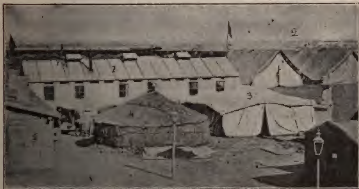
FIG. 209.— Livonian field hospital, Mukden, Manchuria. 1, portable Doecker pavilion; 2, large Russian hospital tents; 3, tortoise tent on ridge pole (system Lefebvre); 4, Mongolian felt tent; 5, small frame barrack for personnel.
